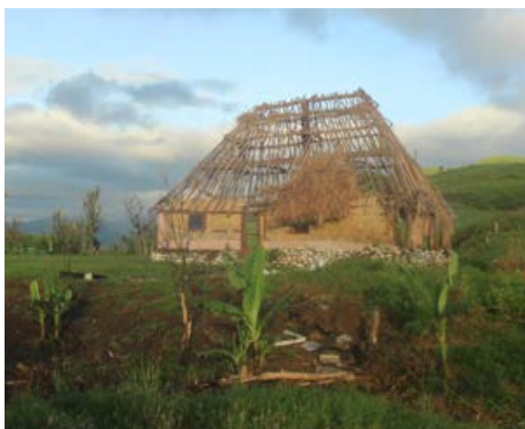
Still standing – a bure, with the thatch blown off; while a nearby school was flattened to the ground.
