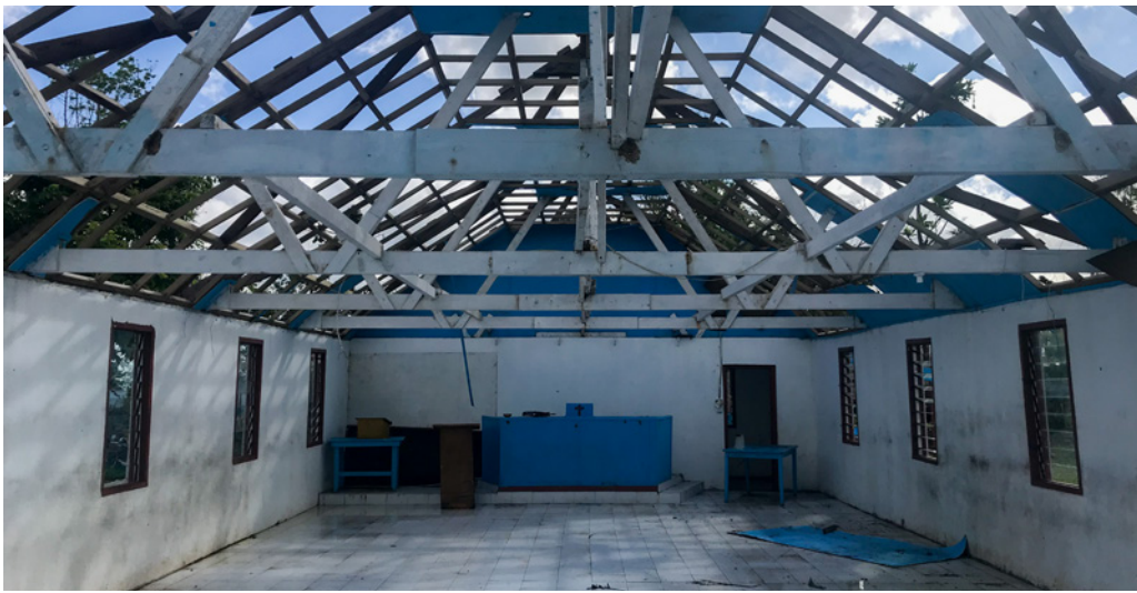
Cyclone Harold damage in Vanuatu.
