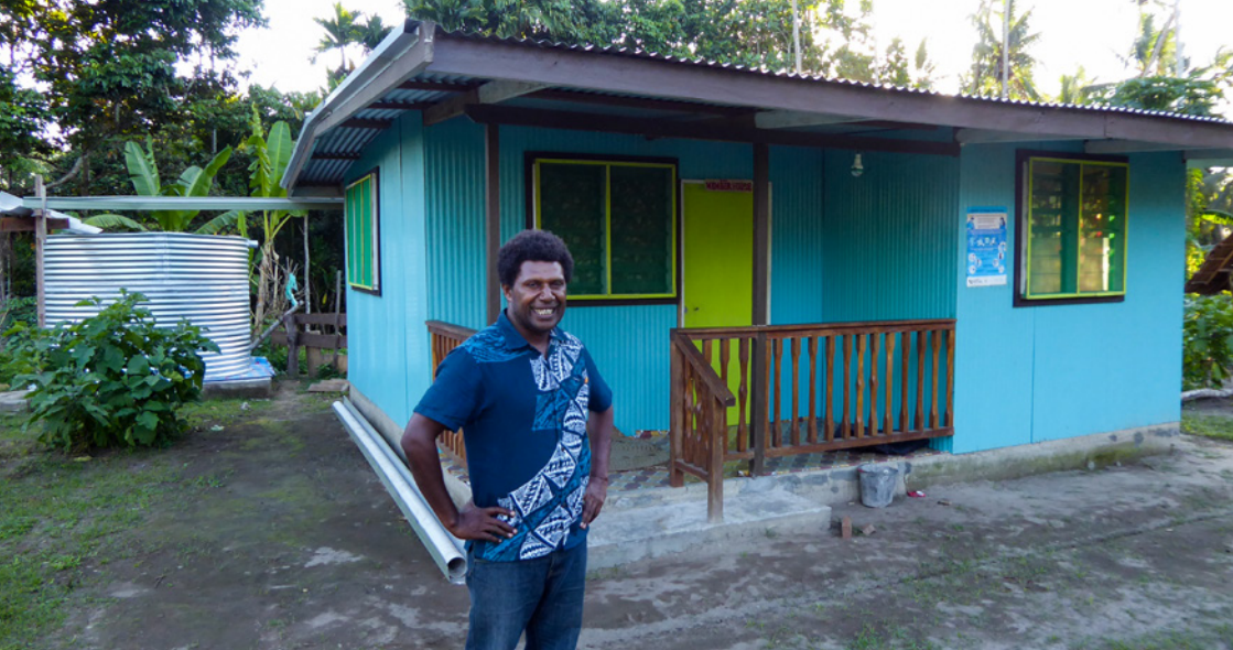
Mr Bauk in front of the newly constructed house for the Ward Officer.
