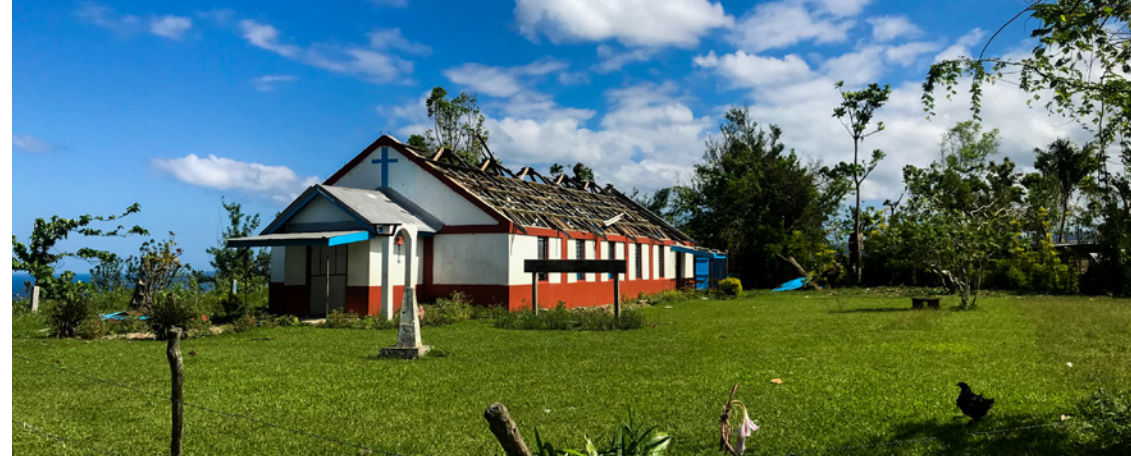
Cyclone Harold damage in Vanuatu.
